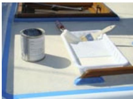
it cannot be kept very long, even in a closed container. We were able to mix enough to cover all of the decks on the first pass. The primer has a consistency a little thicker than milk, and only a light coat was needed. This was easily applied using a small paint tray and a 4-inch foam brush. Once done, the primer needs a 24-hour drying period,
