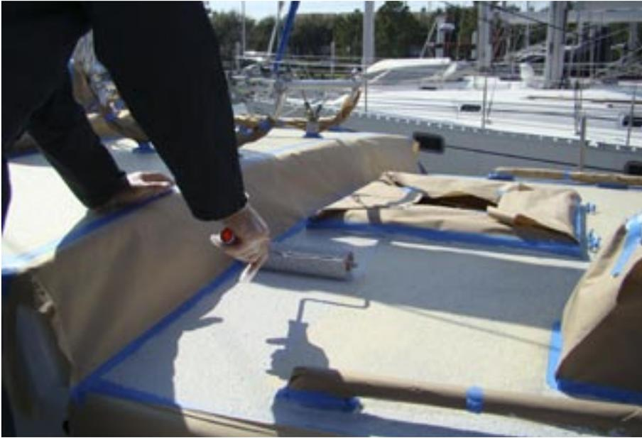
Chuck applies the first of the needed two coats of non-skid with a roller.
